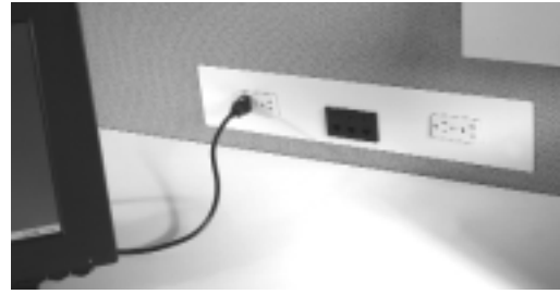
Power panel delivers electrical and data connections at worksurface height.
